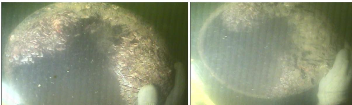
Figure 34. Heavy macrofouling growth in the discharge diffuser piping (diameter of 12 inches).
