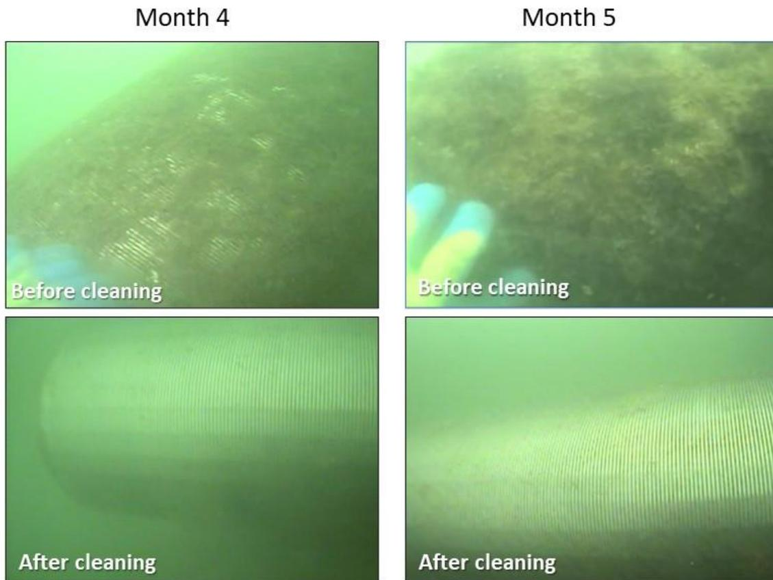
**Figure 22. Photos of the passive WWS before and after external cleaning by divers during months 4 (April 2021 dive survey) and 5 (May 2021 dive survey) of Q2.**
