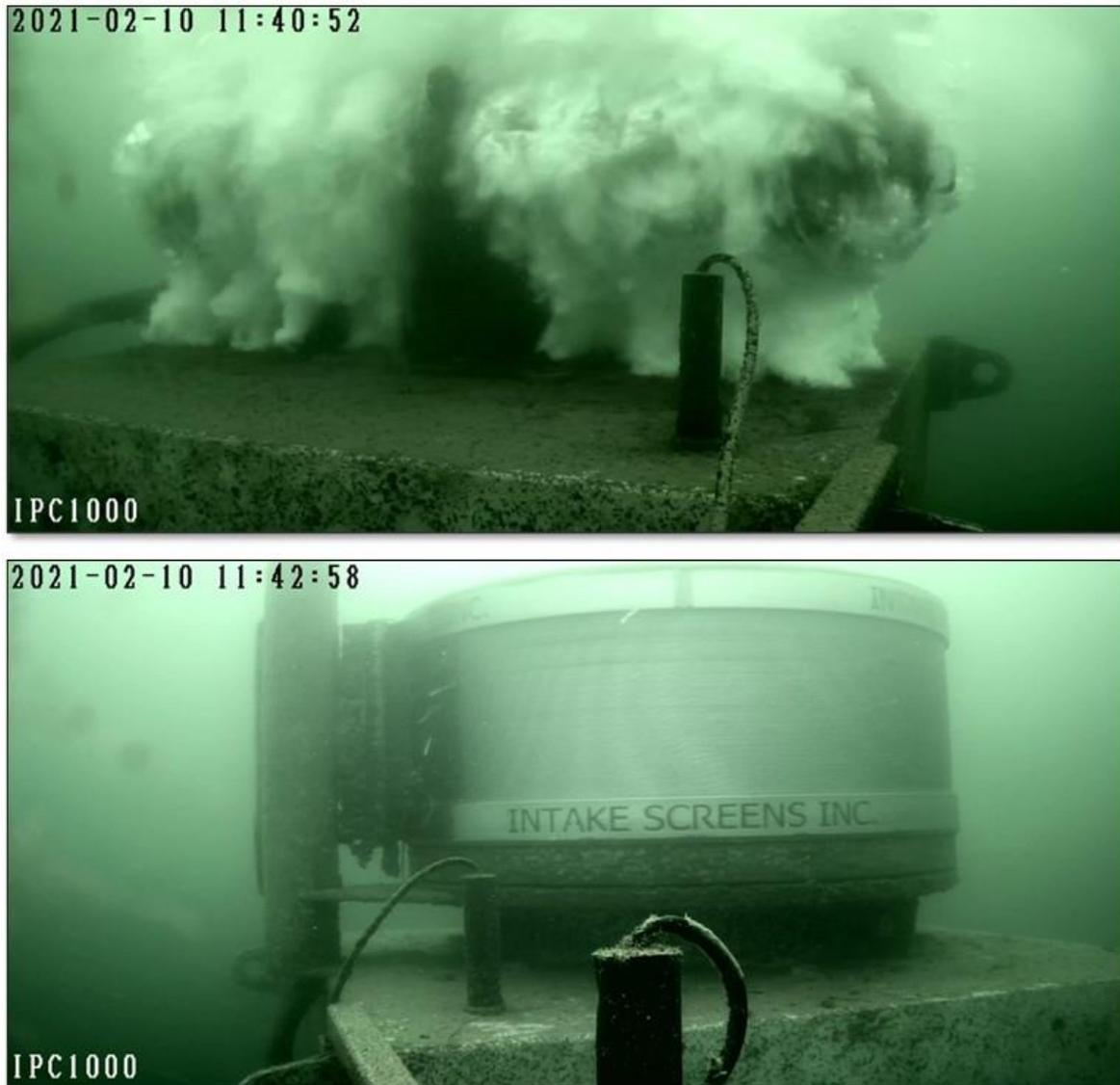
**Figure 4. View of passive wedgewire screen during an airburst (top) and active wedgewire screen (bottom) from submersible, self-cleaning camera during Q1.**
