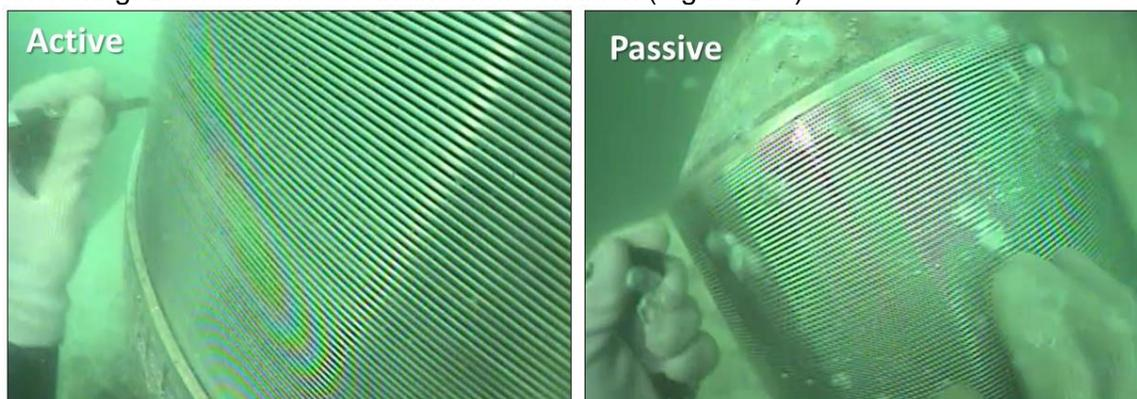
**Figure D-7. Like-new condition of external screening surfaces of active screen (left) and passive screen (right).**
