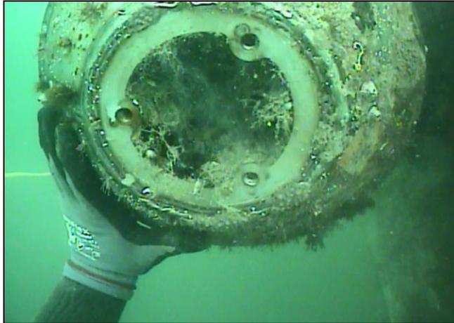
**Figure D-2. Diver photo of fouling inside of passive screen – endcap removed.**
