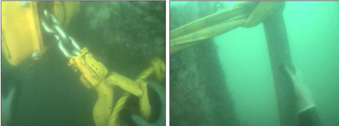
**Figure D-4. Bent anchor clamps on active side being straightened with come-along (left) and using helical anchor shaft for leverage (right)**
