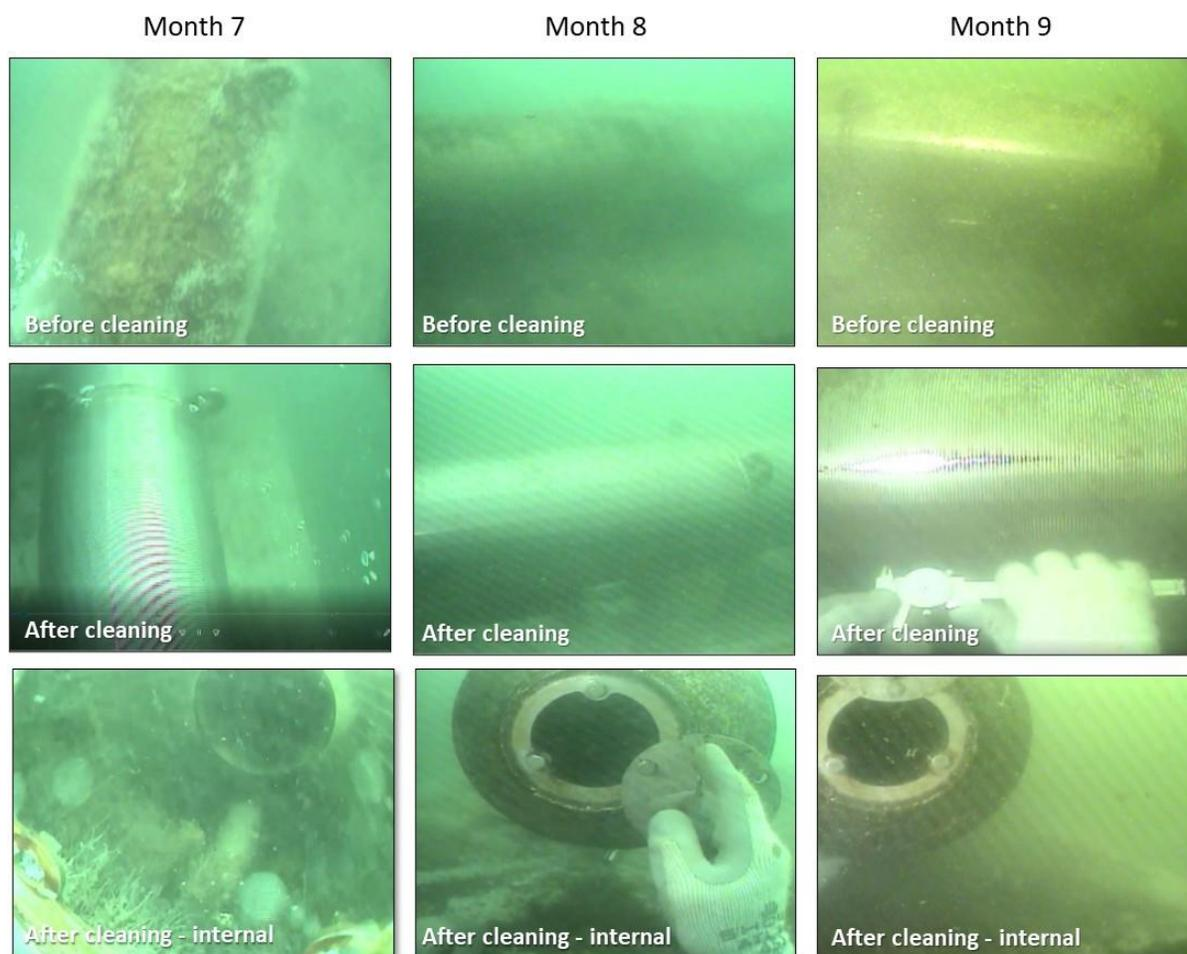
**Figure 26. Photos of the passive WWS before and after external and internal cleaning by divers during months 7 (September 2021 dive survey), 8 (October 2021 dive survey), and 9 (November 2021 dive survey) of Q3.**
