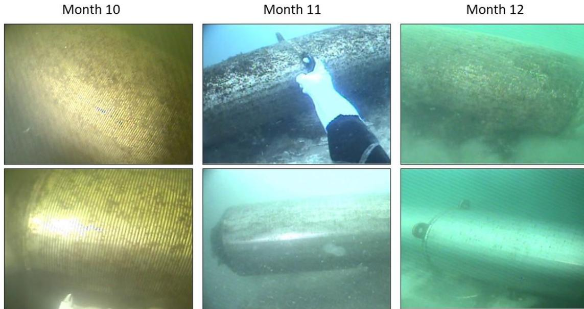
**Figure 31. Photos of the passive WWS before and after external and internal cleaning by divers during months 10 (December 2021 dive survey), 11 (January 2022 dive survey), and 12 (February 2022 dive survey) of Q4.**
