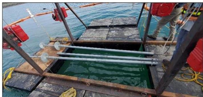
**Figure D-5. One of the two bent active side helical anchors removed (left) and two of the four new helical anchors installed.**
