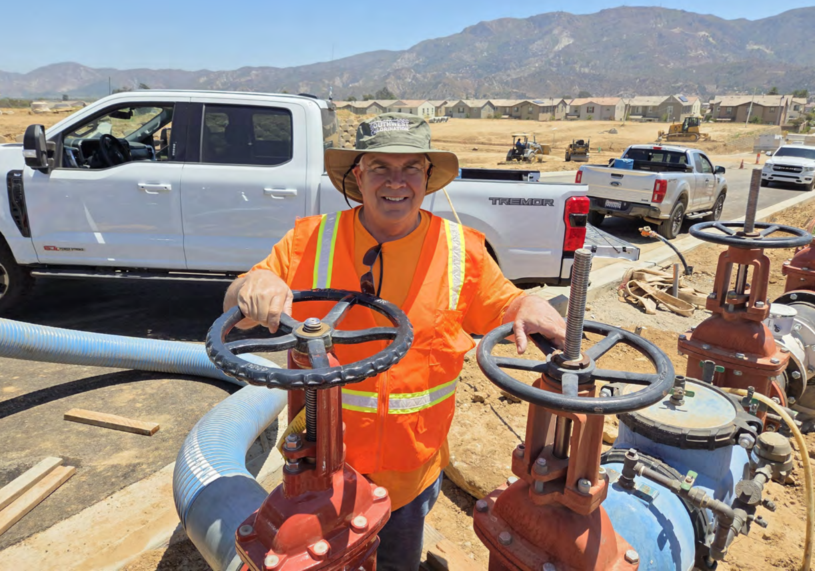
Small business contractor Bill Holmes
