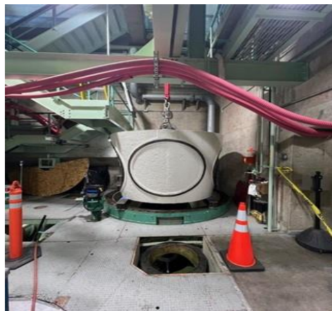
Discharge plug being installed after coating at Iron Mountain.
