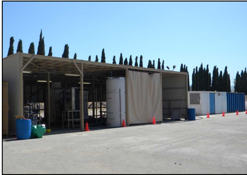
Figure 1-2. Pilot Plant Test Area
