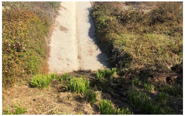
**Photograph 2.** Surface water seeping from beneath v-ditch into Basin 1, facing northeast.
