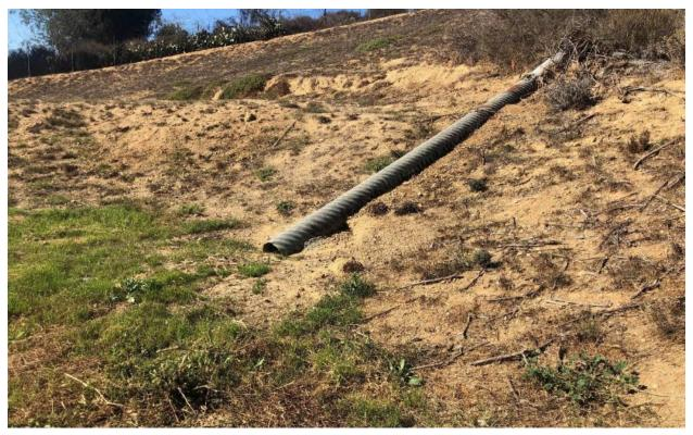
**Photograph 3.** Corrugated pipe conveying runoff into Basin 1, facing west.
