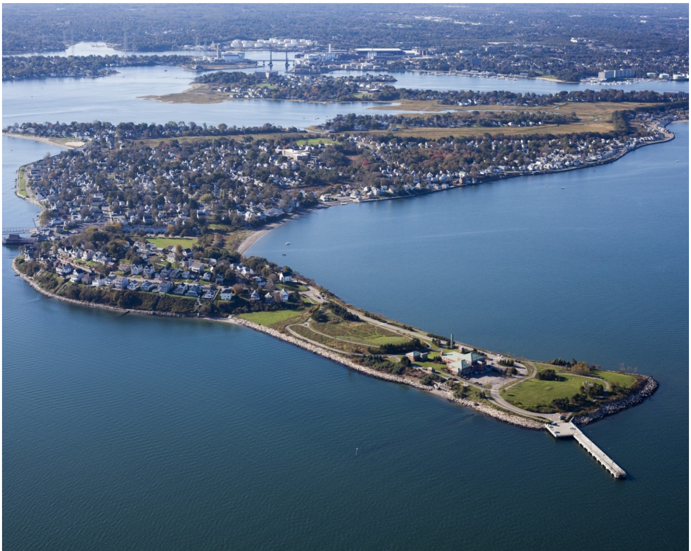
Nut Island Headworks
