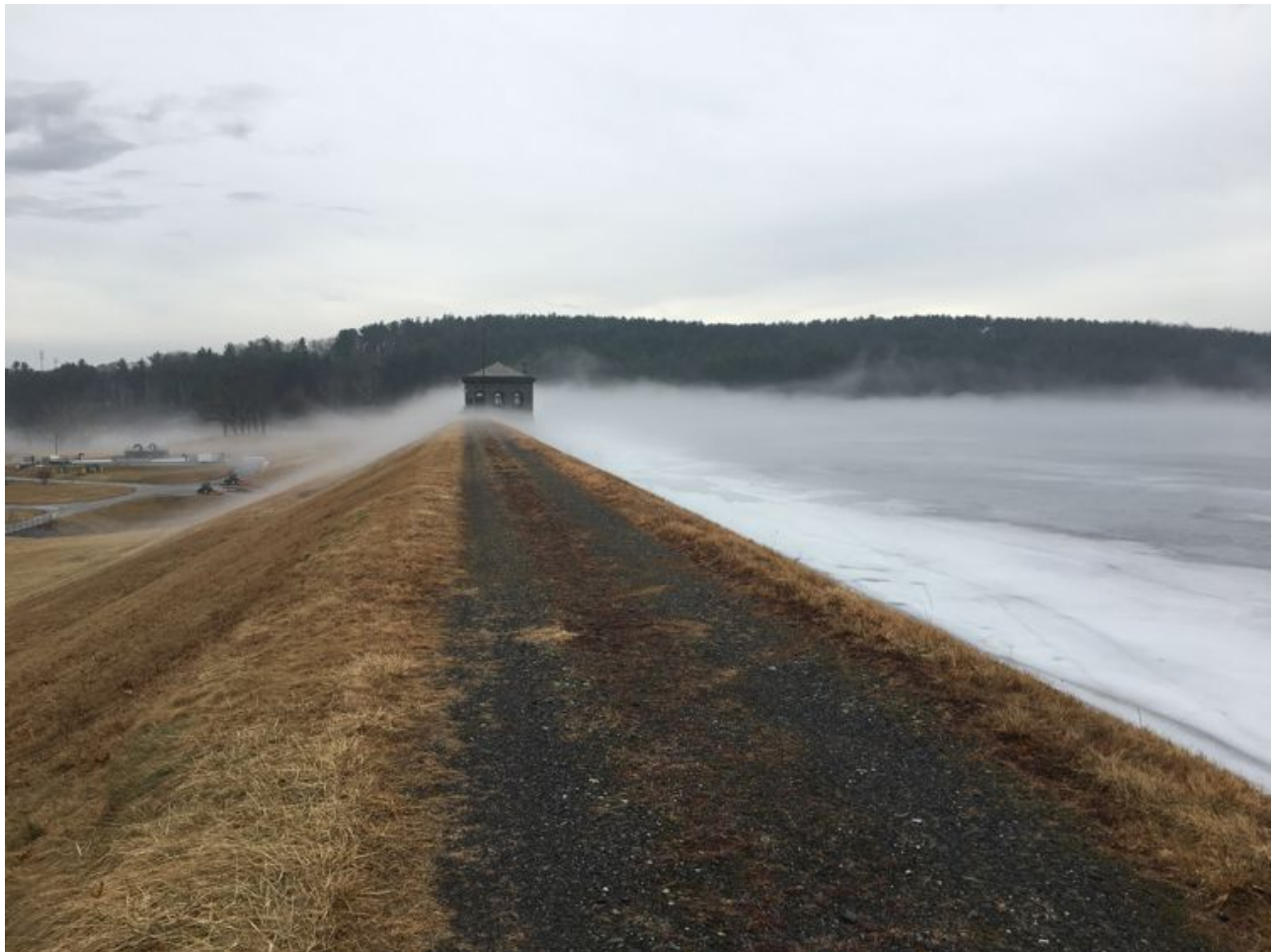
Fog creeping in over Sudbury Dam
