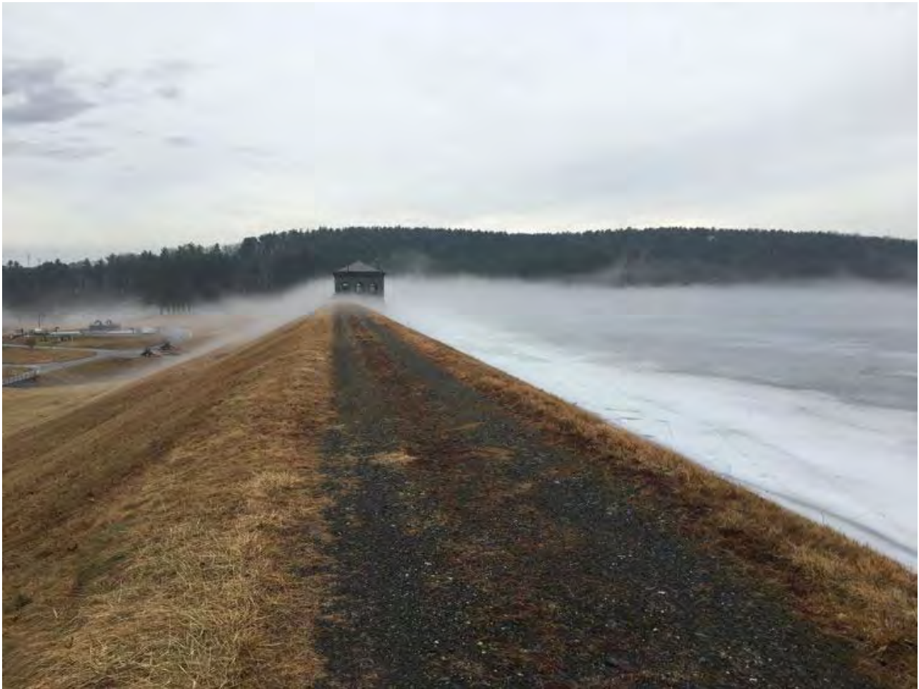
Fog creeping in over Sudbury Dam
