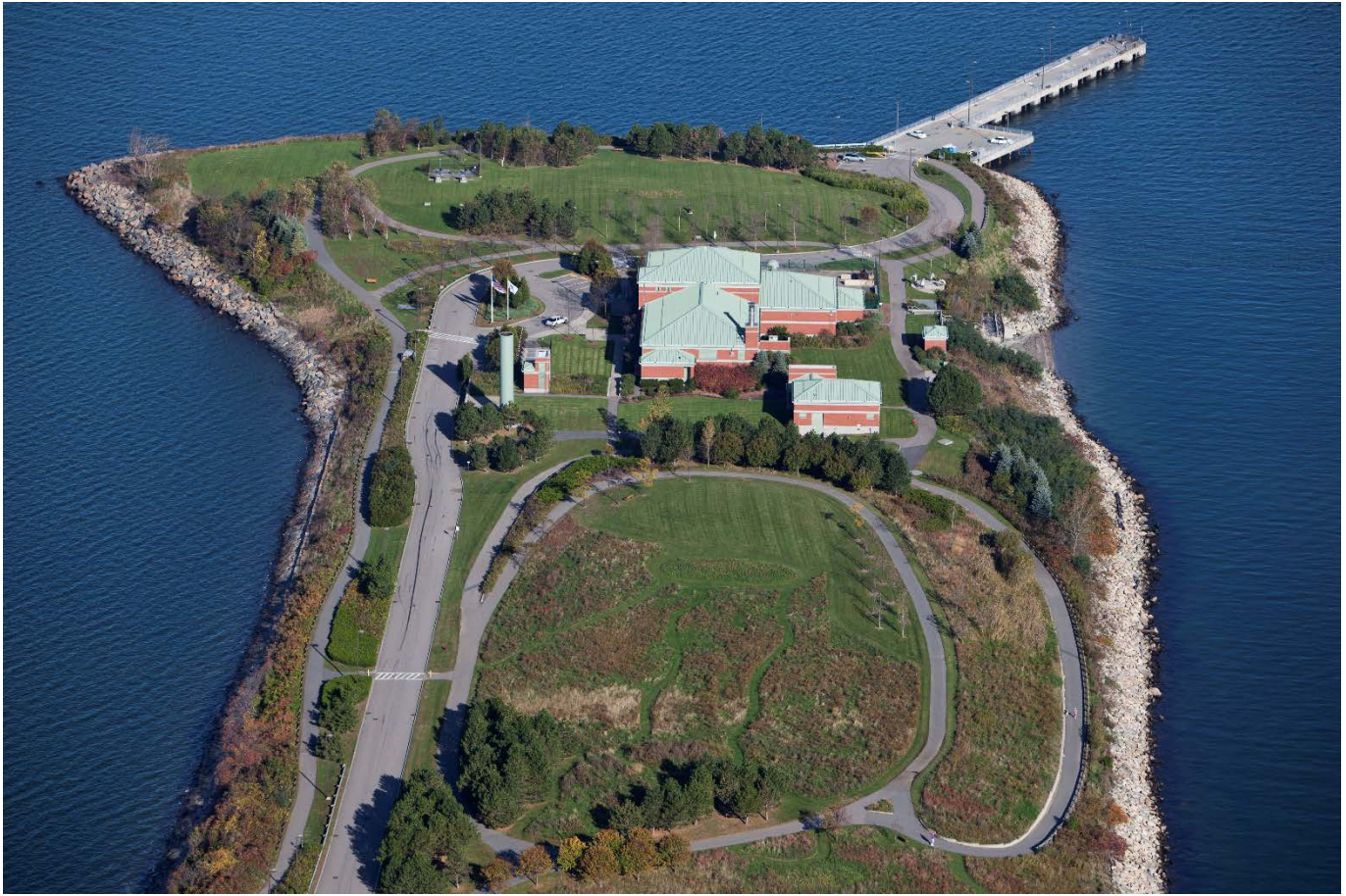
Nut Island Headworks
