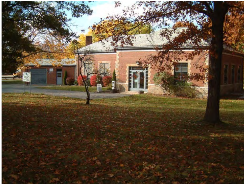
Alewife Brook Wastewater Pump Station
