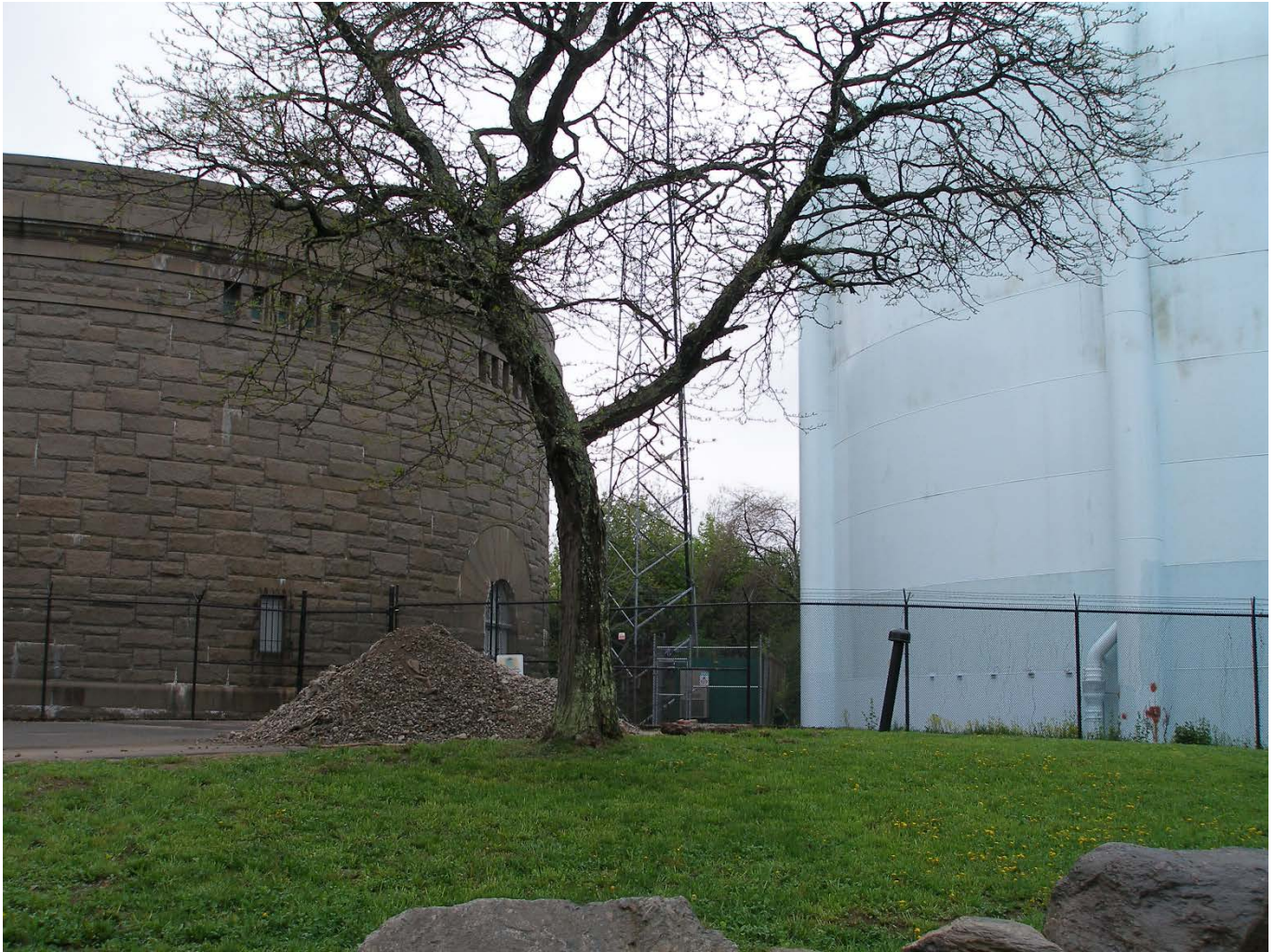
Bellevue Storage Tanks
