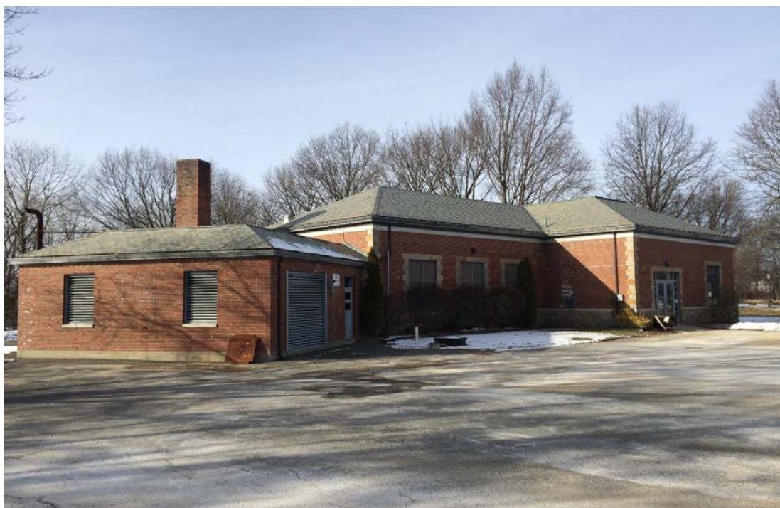
Alewife Brook Wastewater Pump Station
