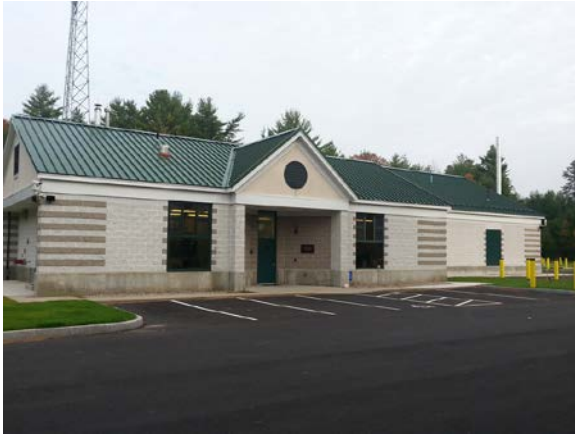
Brutsch Water Treatment Facility
