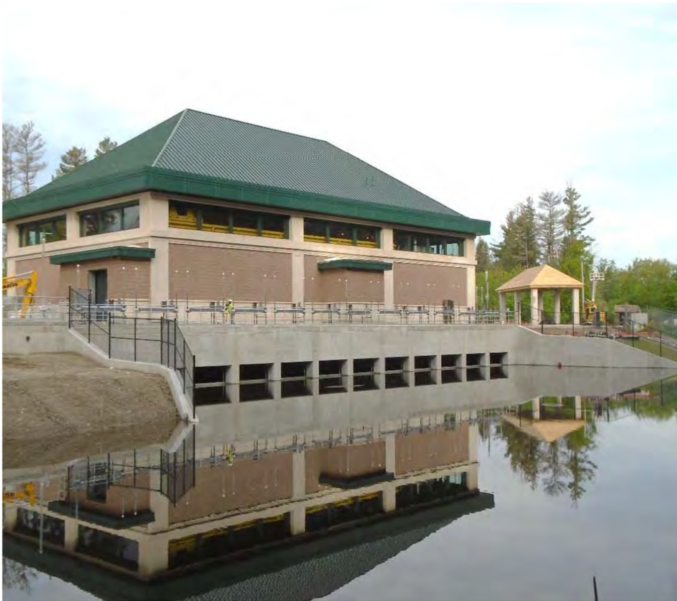
Wachusett Aqueduct Water Pump Station Forebay
