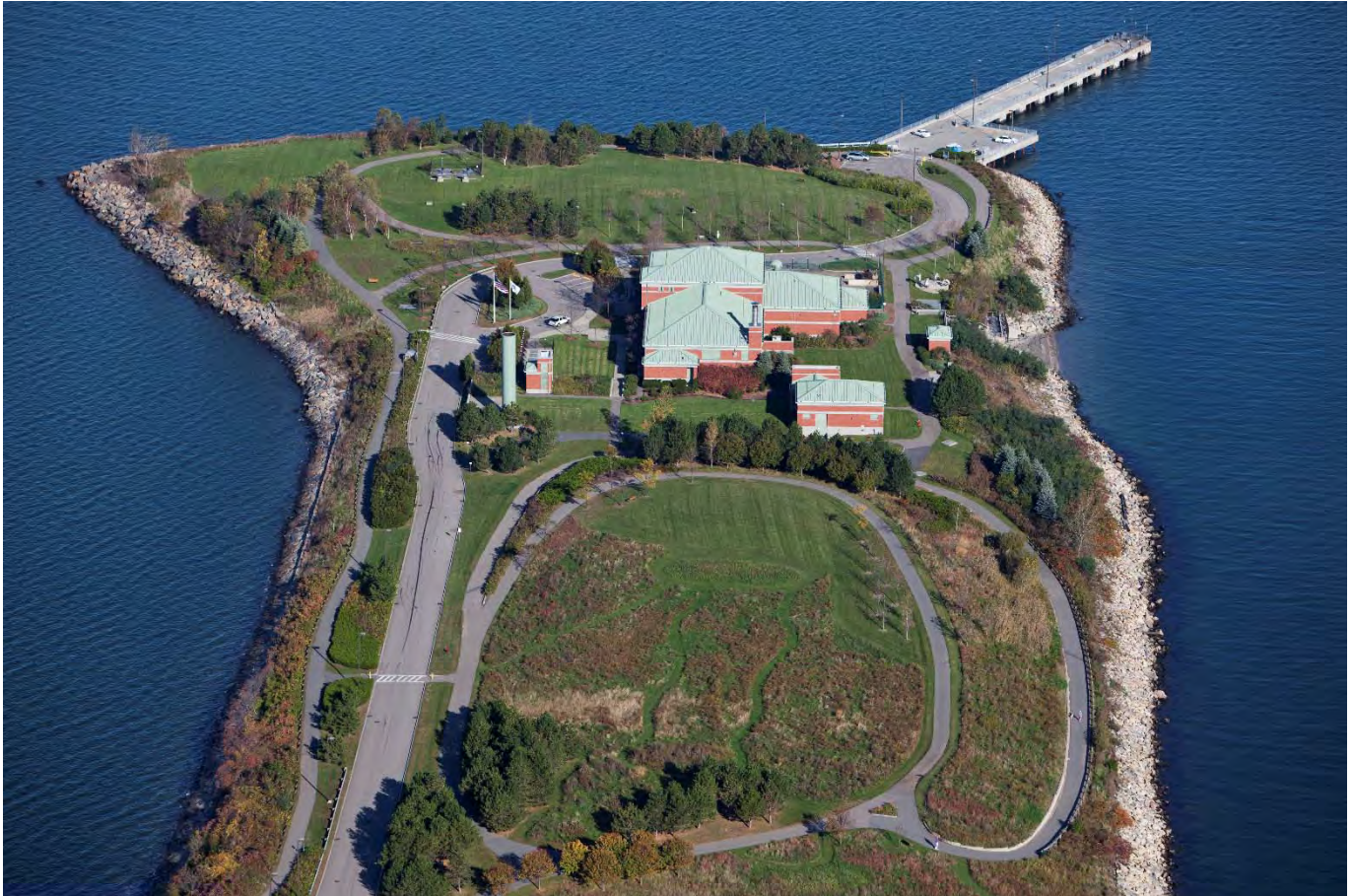
Nut Island Headworks
