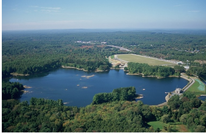
Norumbega Covered Storage Tank
