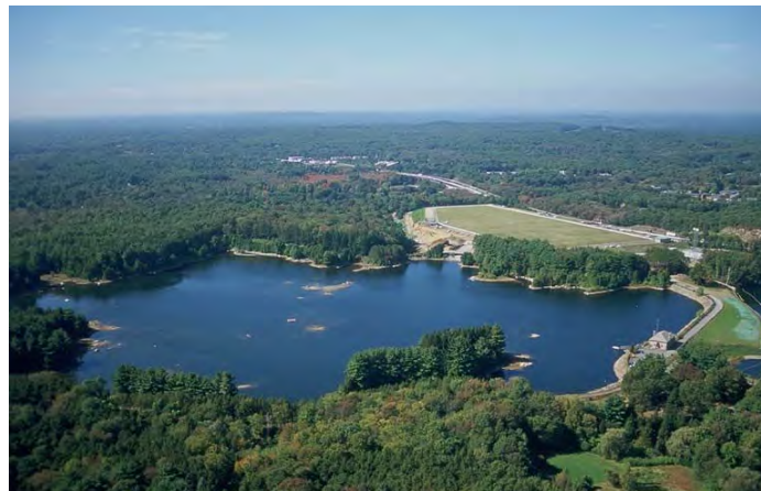
Norumbega Covered Storage Tank
