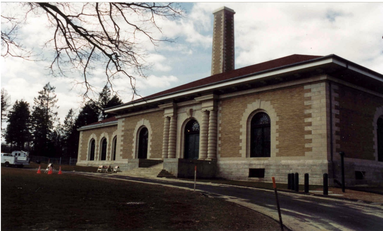
Gillis Water Pump Station
