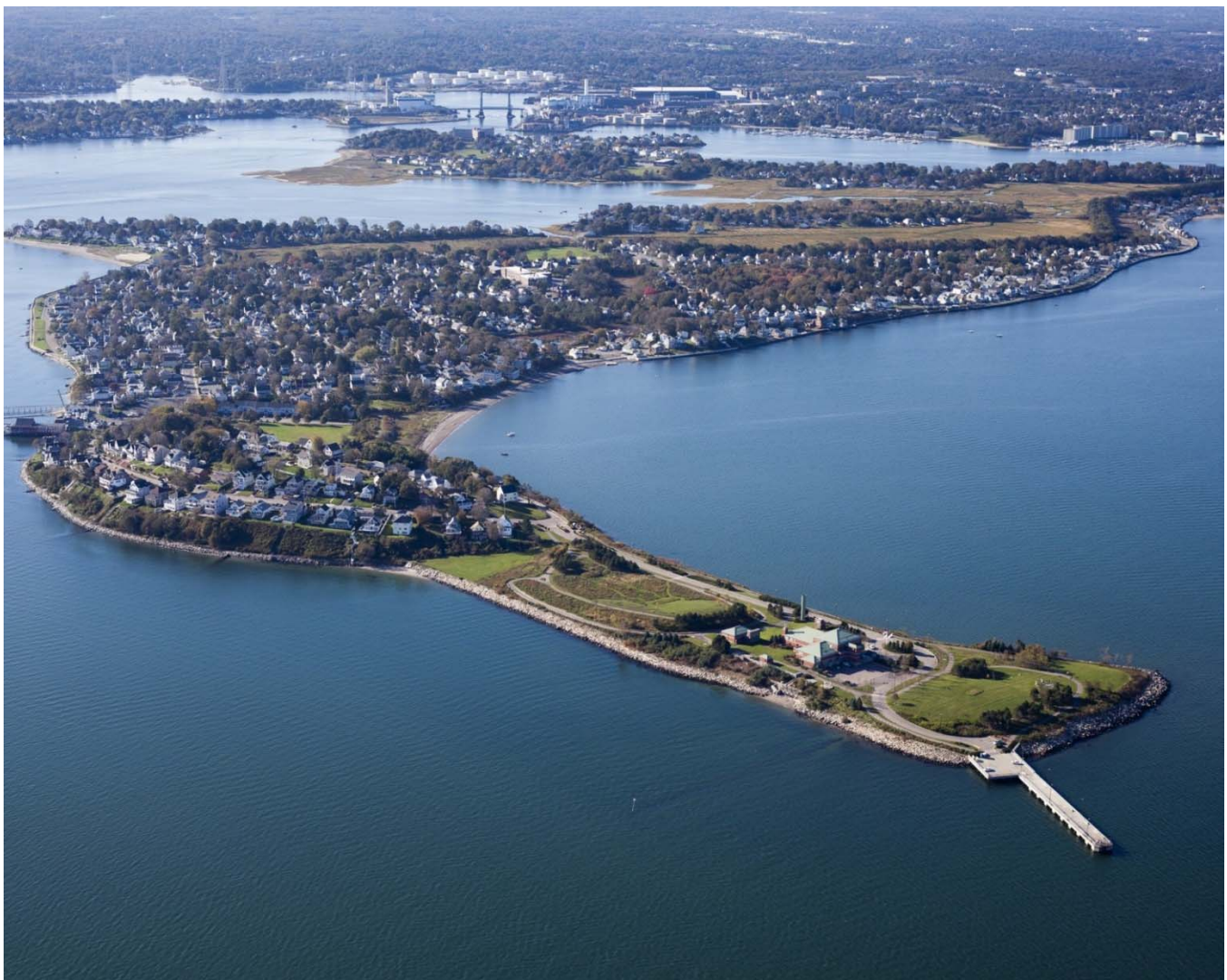
Nut Island Headworks
