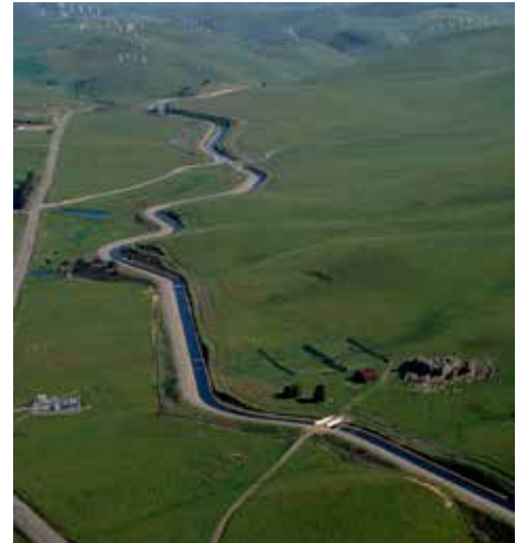
South Bay Aqueduct
