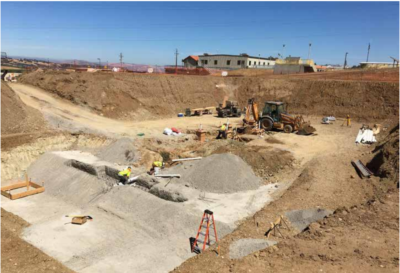
Del Valle Water Treatment Plant Ozone Project
