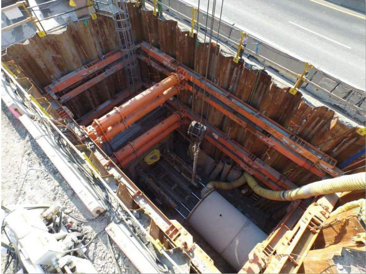
**Figure 3-13** Pipe Jacking from a Rectangular Shaft, [ConstructionEquipmentGuide.com](http://ConstructionEquipmentGuide.com)
