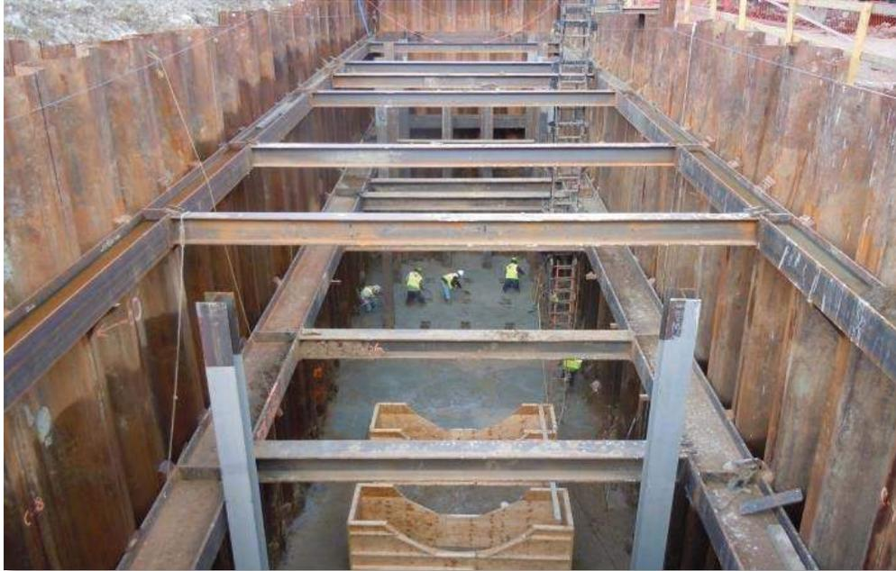
**Figure 3-9 Sheet Pile Excavation Support System, Black & Veatch**
