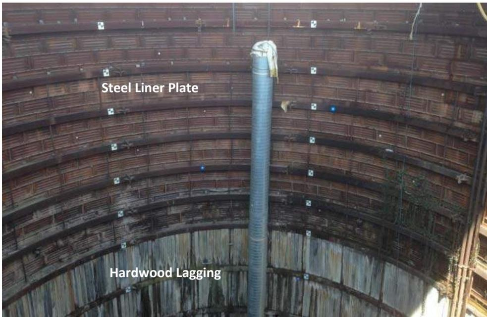
**Figure 3-10 Steel Ribs with Steel Liner Plate (Top) and Hardwood Lagging (Bottom), Black & Veatch**
