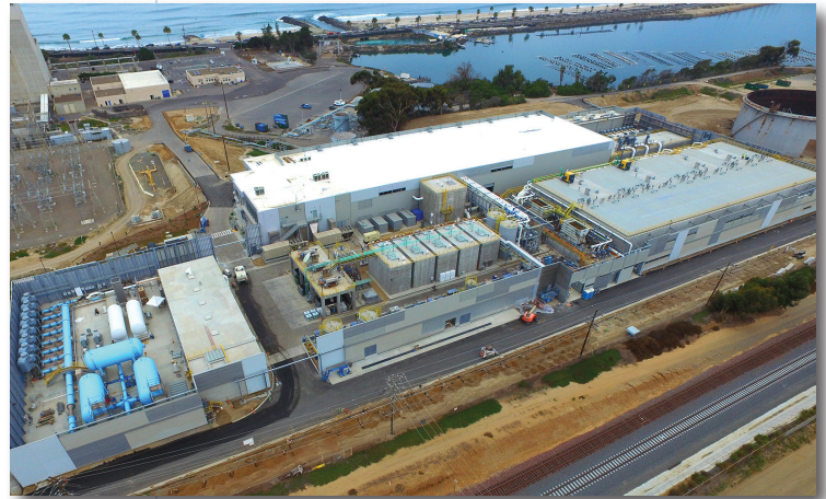
The Claude "Bud" Lewis Carlsbad Desalination Plant started commercial operation in December 2015.
