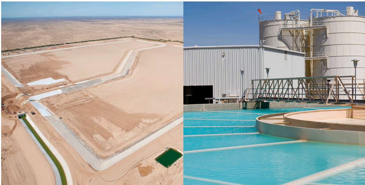
Metropolitan is engaged in a number of projects to maximize Colorado River resources including the Drop 2 Storage Reservoir (pictured left) that captures Colorado River water released from Parker Dam which cannot be delivered to Southern California users for a variety of reasons. In exchange for funding Colorado River system efficiency projects, such as the pilot Yuma Desalting Plant (pictured right), Metropolitan can receive storage credits in Lake Mead which can be drawn on during future dry periods.
