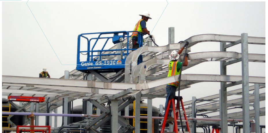
Cable trays being installed at the Regional Recycled Water Advanced Purification Center – a demonstration plant expected to be complete in early 2019.
