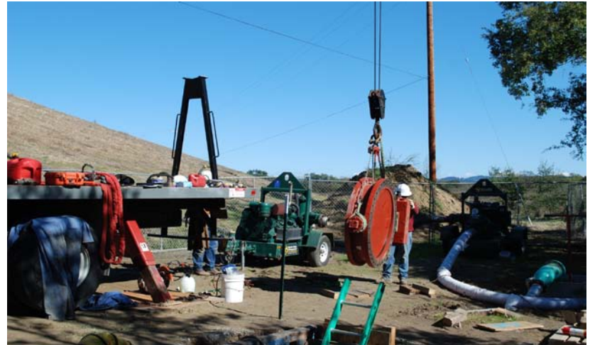
New Butterfly Valve Lowered into Place
