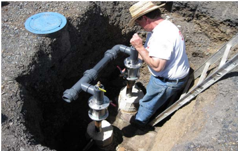
Installing New Upgraded Air Valves
