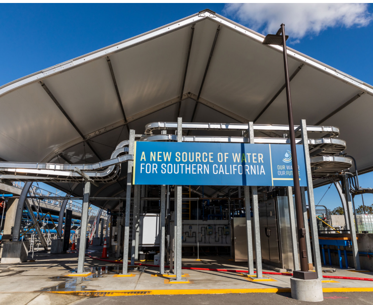
Regional Recycled Water Advanced Purification Center, Carson, California
