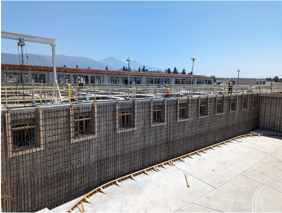
Figure 4-1: Seismic Reinforcement of Weymouth Basin 7
